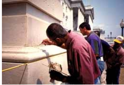
Masons practice using lime putty mortar to repair historic marble. Photo: NPS files.
