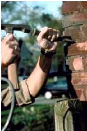
Here, a hammer and chisel are being correctly used to prepare a joint for repointing. Photo: John P. Speweik.
