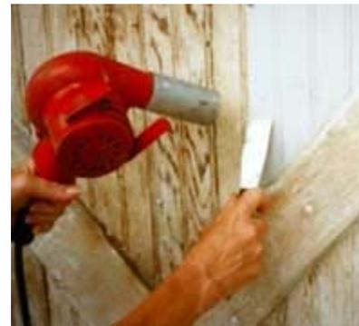
The nozzle on the electric heat gun permits hot air to be aimed into cavities on solid decorative surfaces, such as
