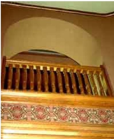
A return air grille is successfully screened behind the arch. Photo: NPS files.
