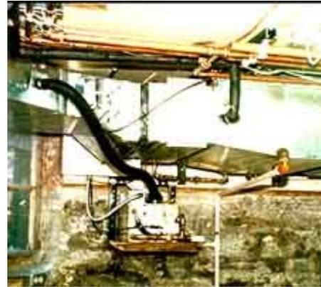
A fan coil unit in the basement is feeding controlled air to a primary space upstairs.
