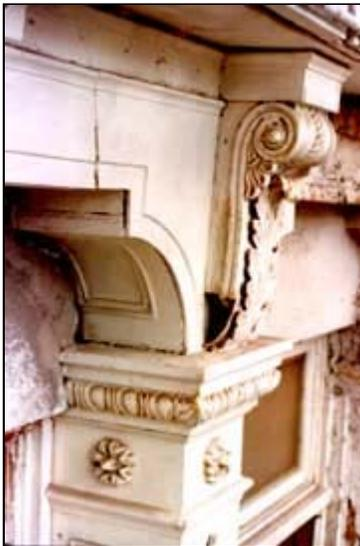
Structural crack, gaps at joints between components, and a large opening where part of the console bracket is missing are the problems evident in this cast-iron assembly. Photo: Ford, Powell & Carson.
