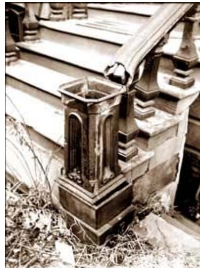
architectural element causes rust that may streak down over other architectural elements. The water may freeze, causing the ice to crack the cast iron. Cracks reduce the strength of the total cast iron assembly and provide another point of entry for water. Thus, it is important that cracks be made weathertight by using caulks or fillers, depending on the width of the crack.
