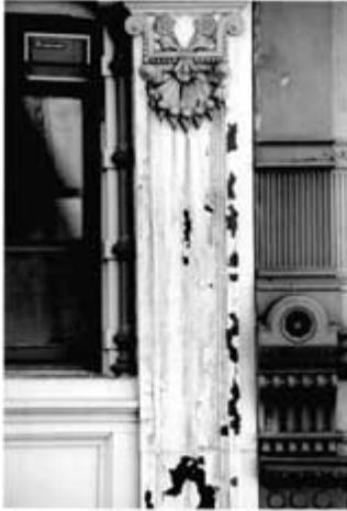
On this building, a strong alkaline paint remover was used, and apparently was not adequately rinsed or neutralized. Over a period of months, the newly applied paint began to peel and streaks of rust appeared on the iron. Photo: Kim Lovejoy.
