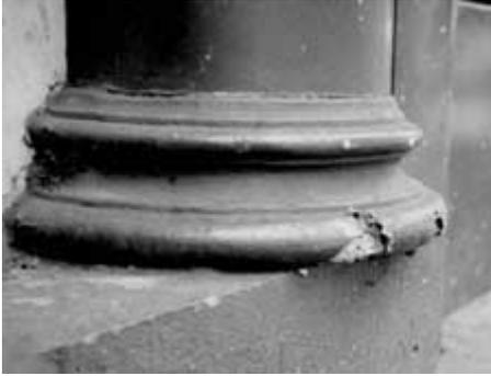
This lightweight fiberglass column at street level sustained damage from impact within a few years of installation. Photo: Building Conservation Associates.
