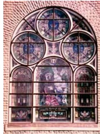
The grid for this protective glazing disregards the configuration of the historic window. The new framing system also causes distracting shadows on the interior. Photo: Neal A. Vogel.
