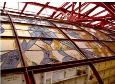
Before repairs began on the vaulted glass ceiling, a new diffusing skylight was installed to correct
