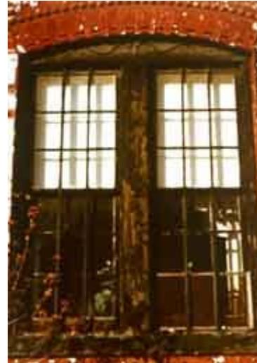
Deteriorating operable windows often contribute to lead dust in a house. In homes with small children, floors and other surfaces should be kept as clean as possible to avoid lead contamination.
