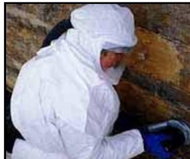
**Lead-based paint, a toxic material, was widely used in North America on both the exteriors and interiors of buildings** until well into the second half of the twentieth century. If a "historic" place is broadly defined in terms of time as having attained an age of fifty years, this means that almost every historic house contains some lead-based paint. In its deteriorated form, it produces paint chips and lead-laden dust particles that are a known health hazard to both children and adults.
