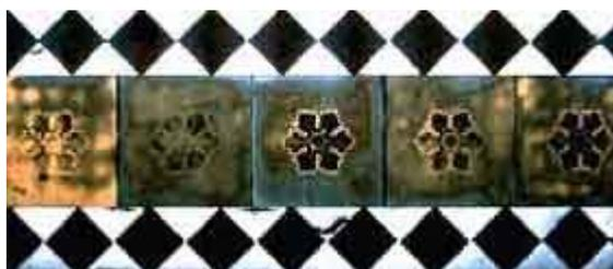
Worn encaustic tiles are still serviceable, but once the design has been lost, the tiles cannot be repaired. They must be replaced in kind, to match. Photo: NPS files.
